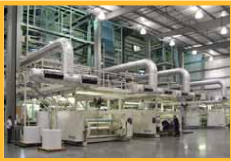
Danafilms' new Franklin, Kentucky state of the art blown film plant.
